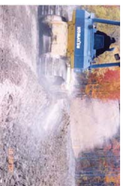
Fig. 12. Moderately dry topsoil is being replaced on the affected site now that Phase 1 deep ripping of the compressed subsoil is complete.
