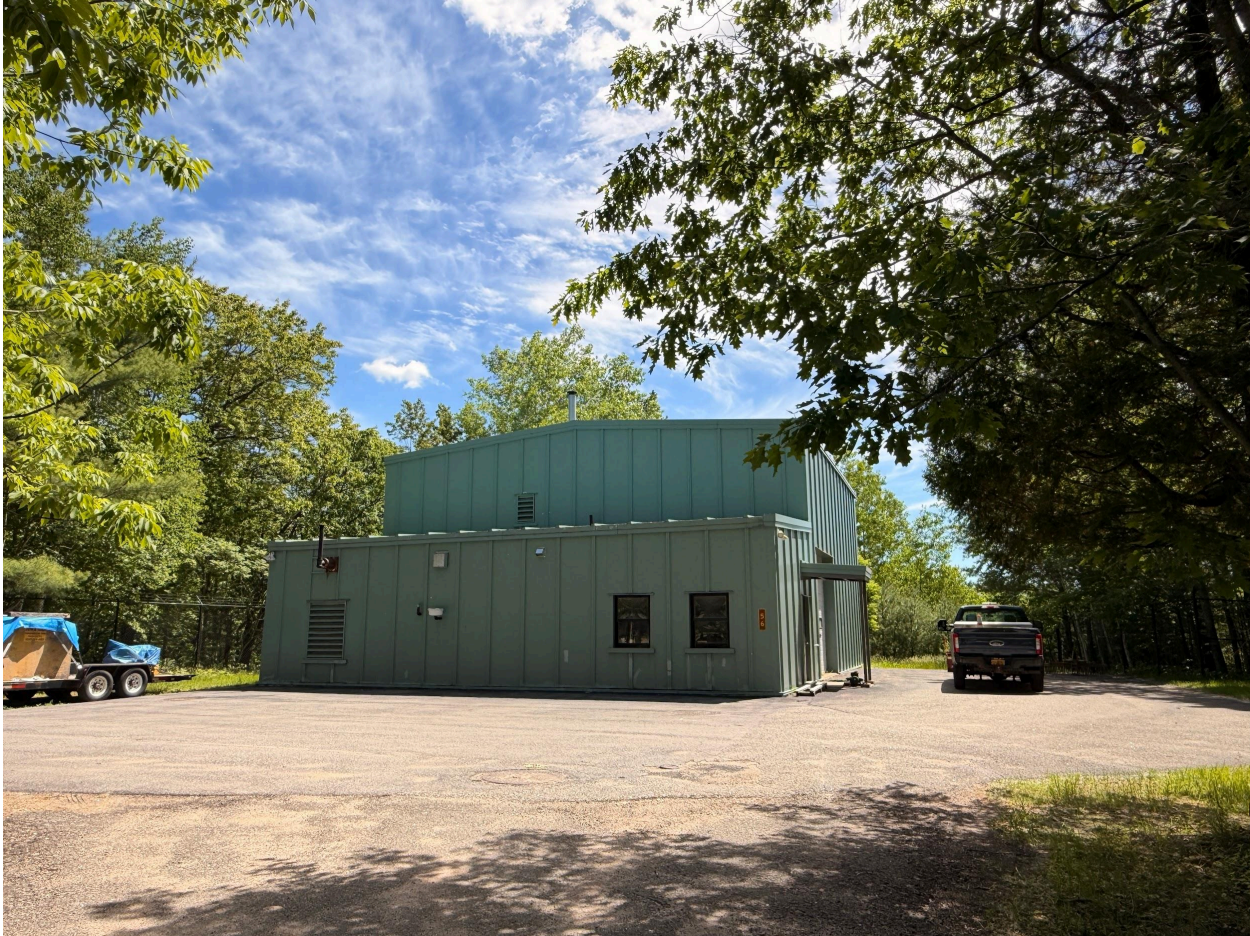
Filtration system building:
