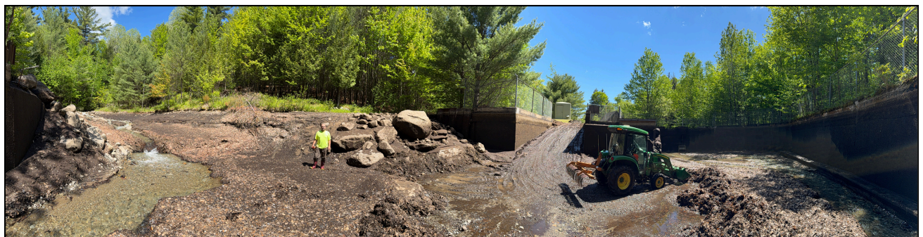
Cleaning out the Whitebrook Water Reservoir
